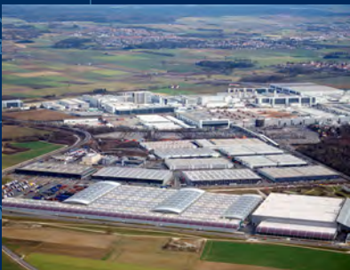
GVZ logistic centre, Germany
