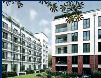
Apartment Building Hamburg, Germany
