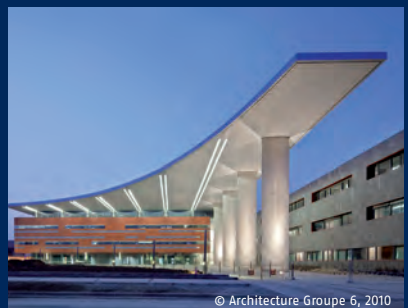
Hospital Clermont-Ferrand, France
