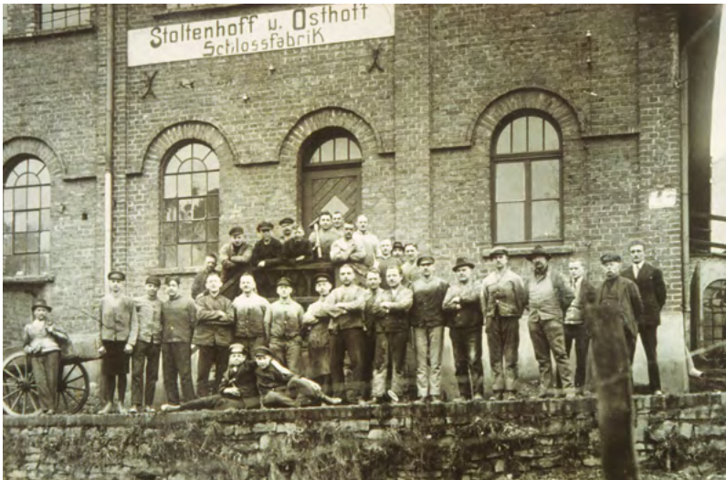
1910s – The building of the local lock factory Stoltenhoff and Osthoff has been owned by ABUS since 1929.
